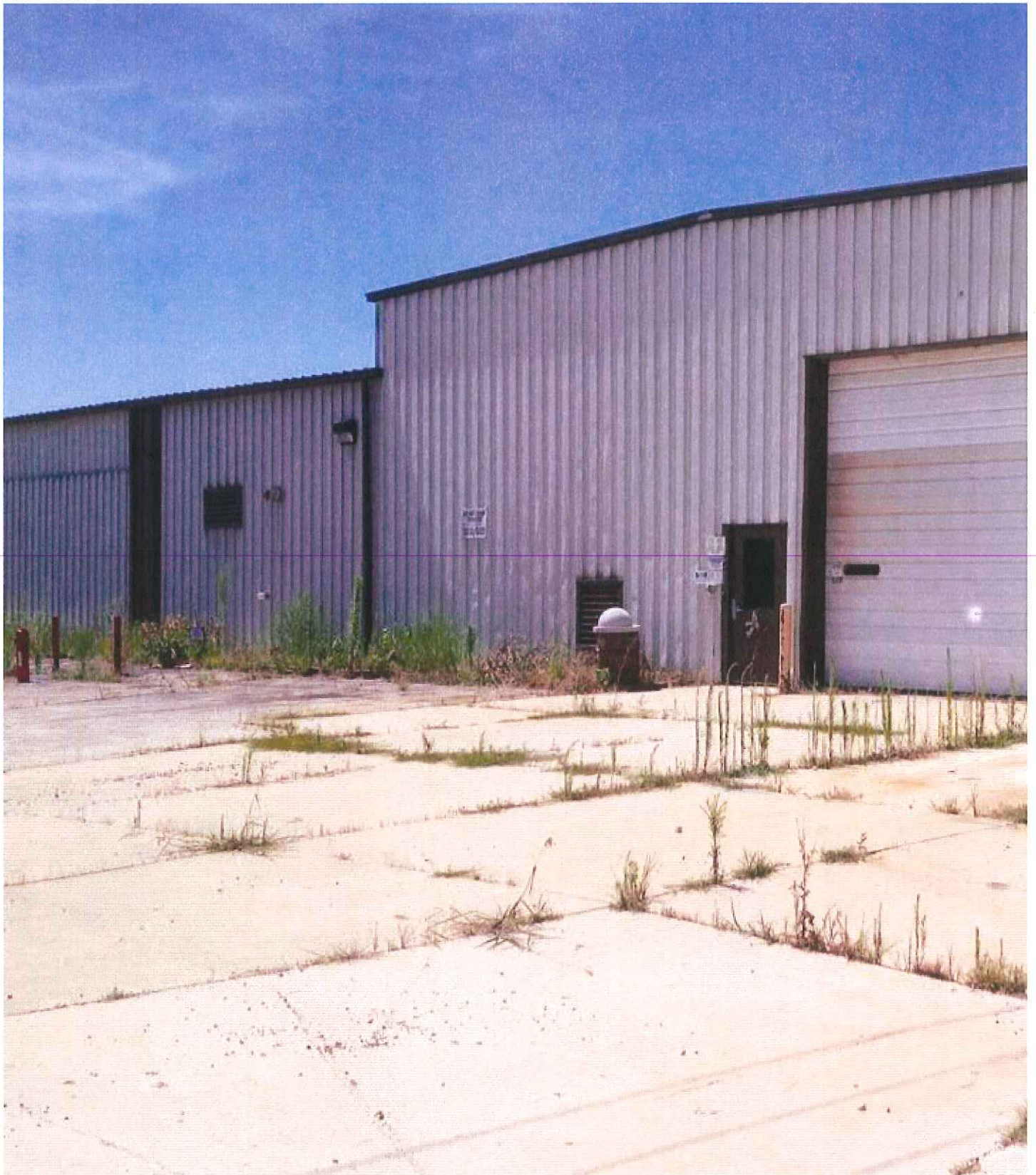
Current Bldg at 326 Industrial Ave. showing existing overhead East & N Doors.
