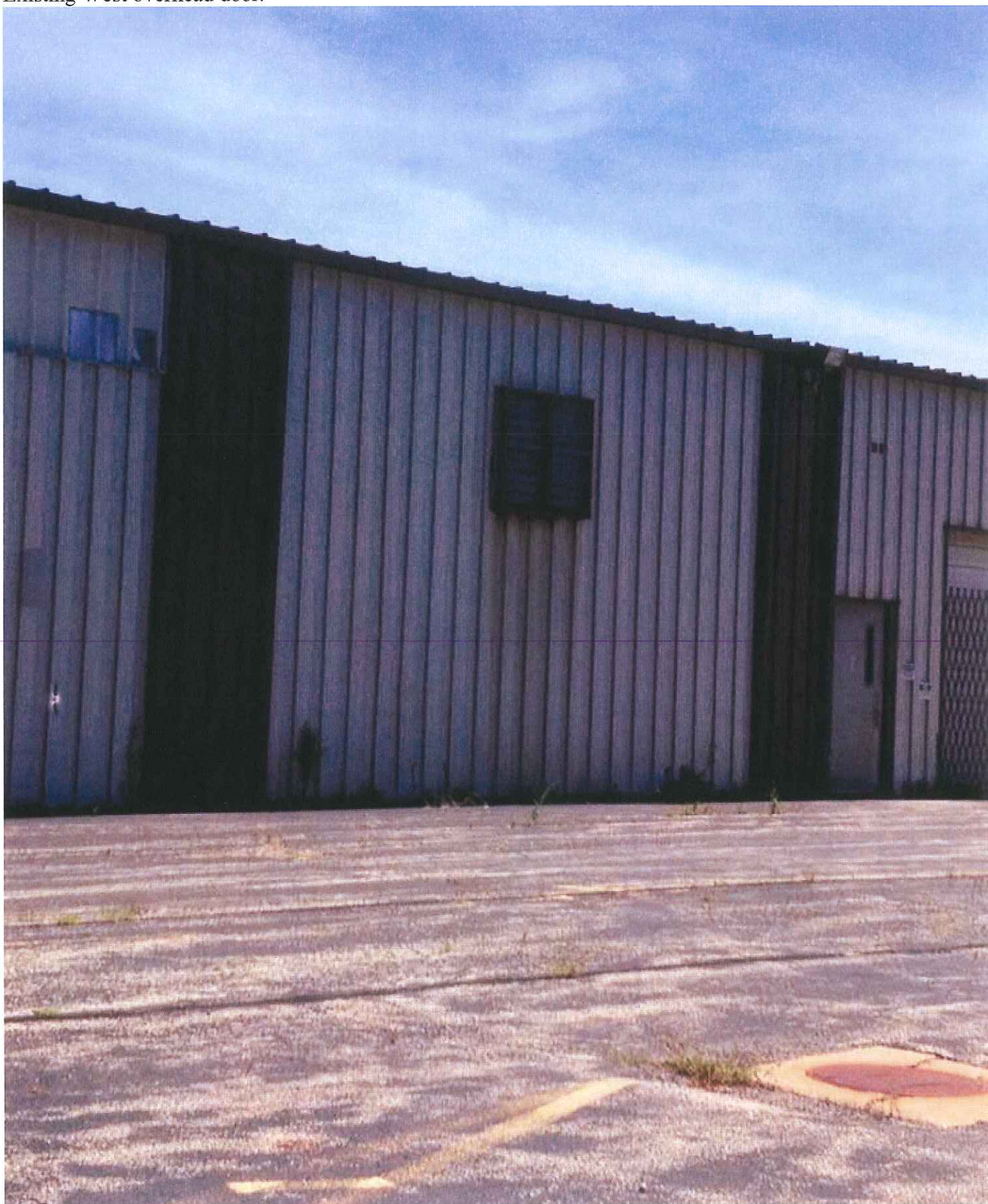
Existing West overhead door.
