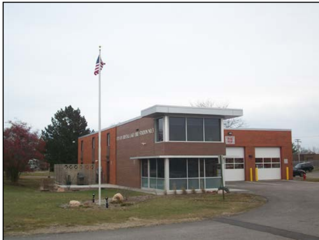
Fire Station Three 844 Virginia Road
