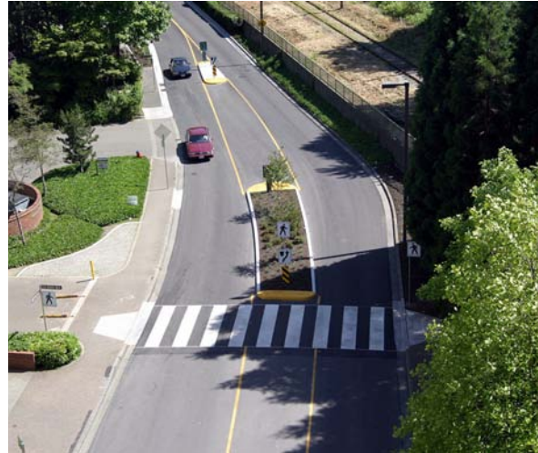
Figure 4.14. Examples of high visibility crosswalks
