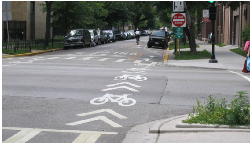
Figure 4.17. Examples of through-intersection bikeway markings
