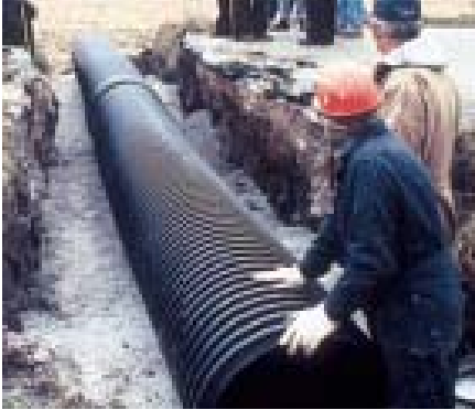
FIGURE T-1 – INSTALLATION OF PERFORATED TILE
