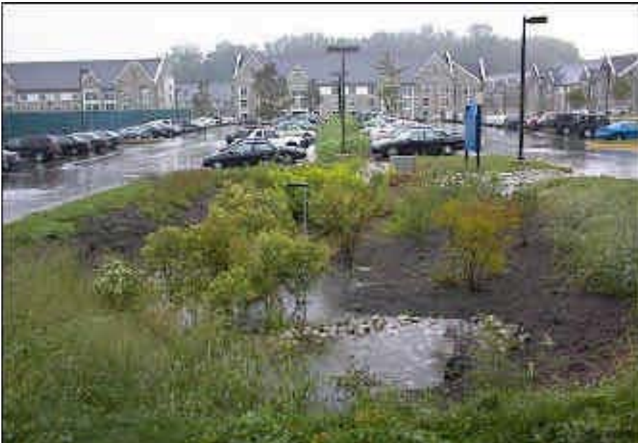
FIGURE SD-2 – BIO-RETENTION ISLANDS
