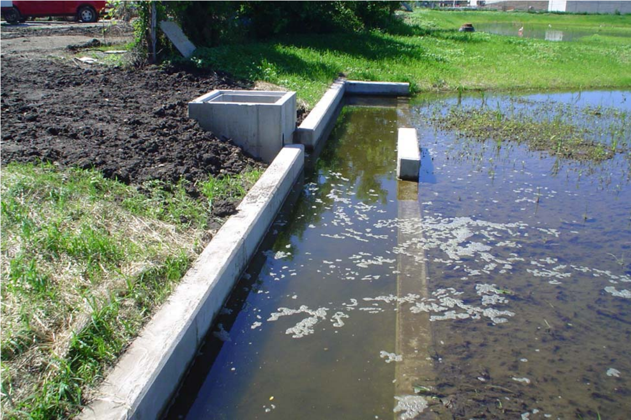
FIGURE WB-4 – LEVEL SPREADER
