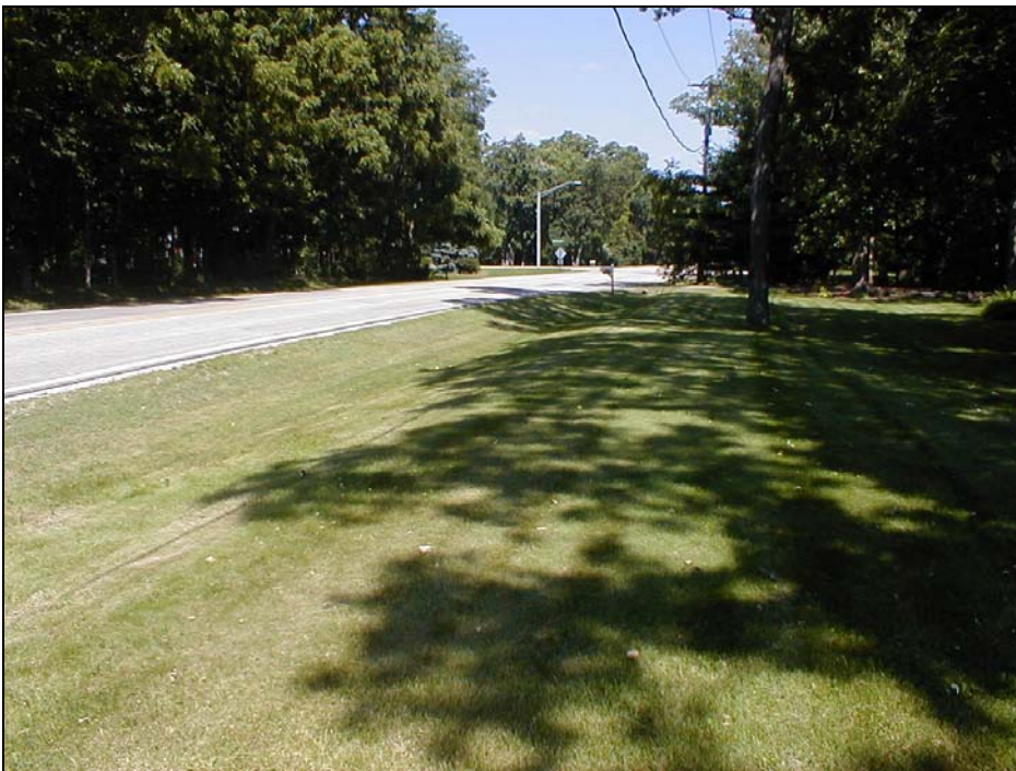
FIGURE SD-4 – VEGETATED SWALE
