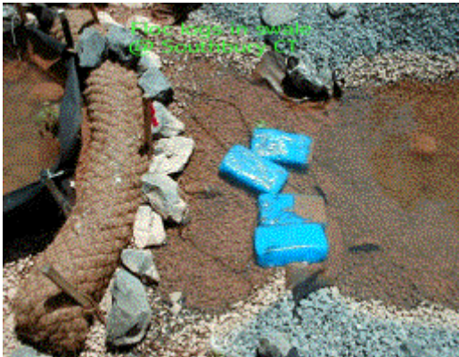
FIGURE EC-2 – FLOC LOG INSTALLATION
