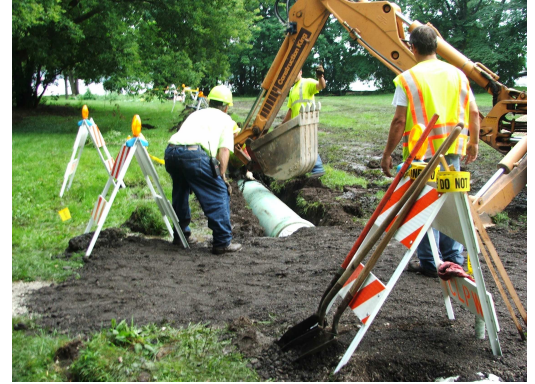
Construction of the North Shore Detour
