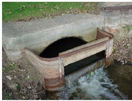
Existing Cove Pond Outfall at Lake
