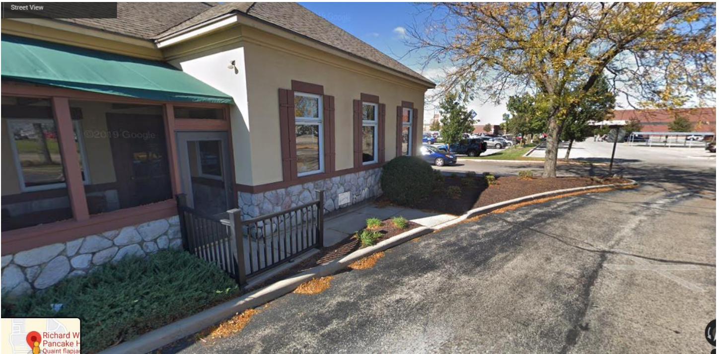
Door which servers would use to access outdoor seating located in the parking lot.
