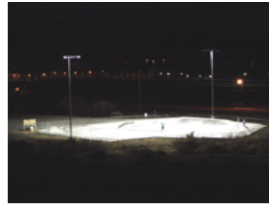
Sports facility USING full-cutoff luminaires
