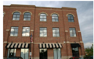
EIFS not permitted as primary material
