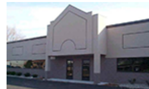
EIFS not permitted as primary material
