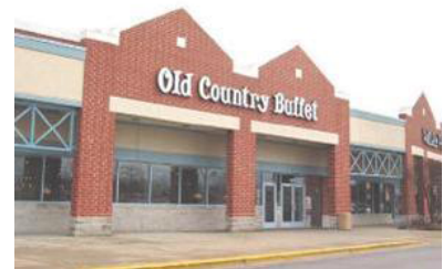
Applied veneer "movie set" storefronts not permitted.
