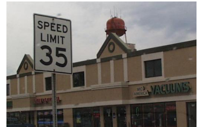
EIFS not permitted as primary material
