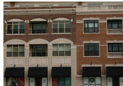
Highlight architectural elements
