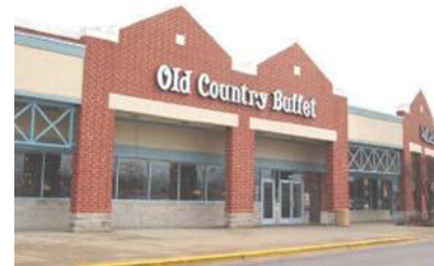
Parapet wall conveying 2-D paper facade is not permitted.
