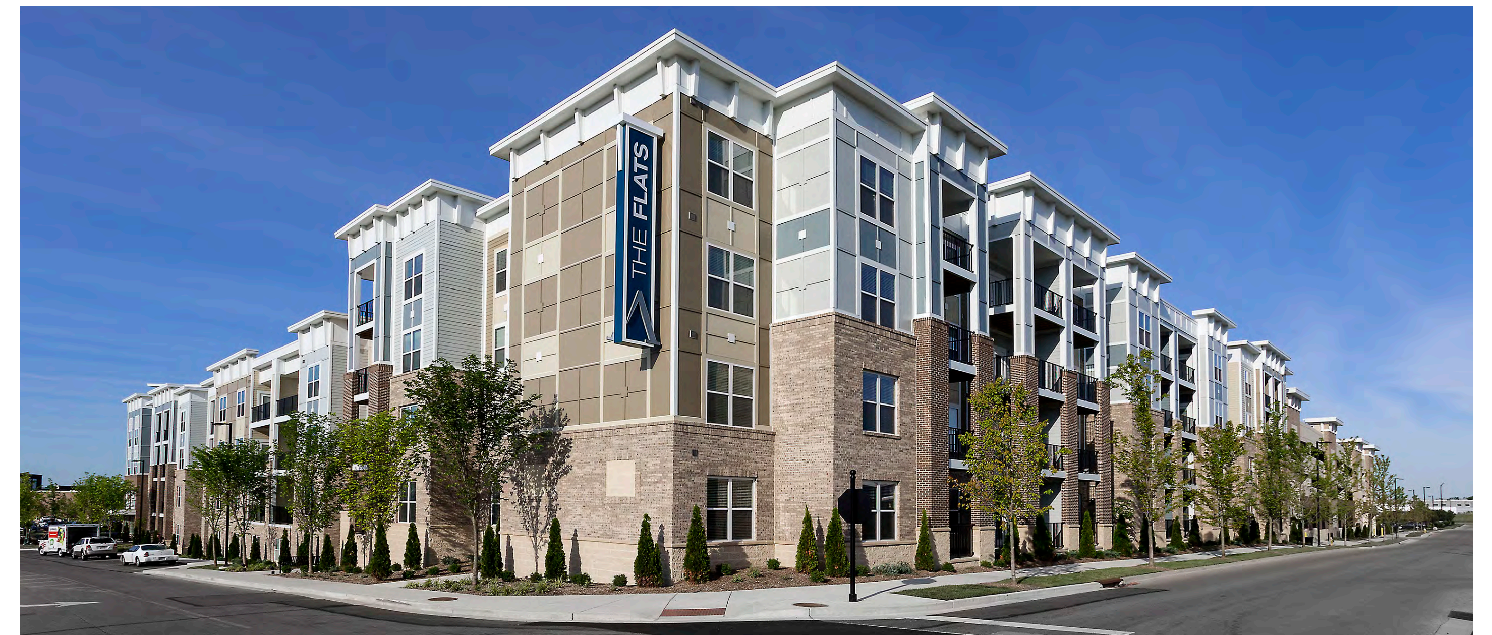
Undulating traditional architectural stacked horizontal and vertical facade elements with a rhythm of a subtle blended palette of paired masonry and cementitious panels
