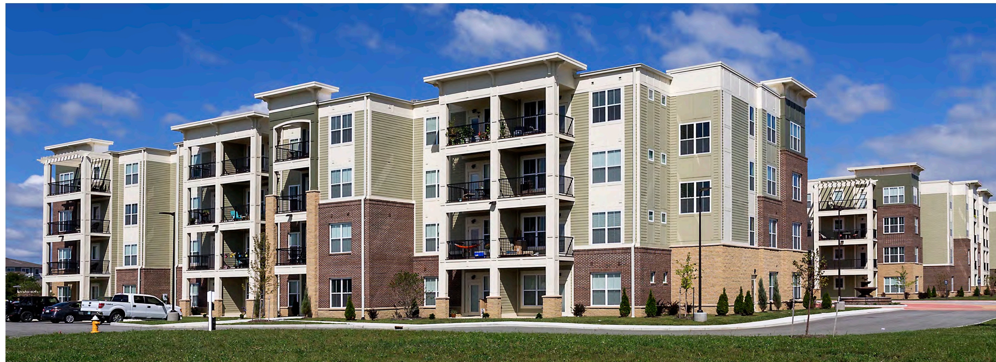
Varied Materials and textures with a multi-level brick base, an articulated cornice line frames vertical elements and enhances the building perimeter
