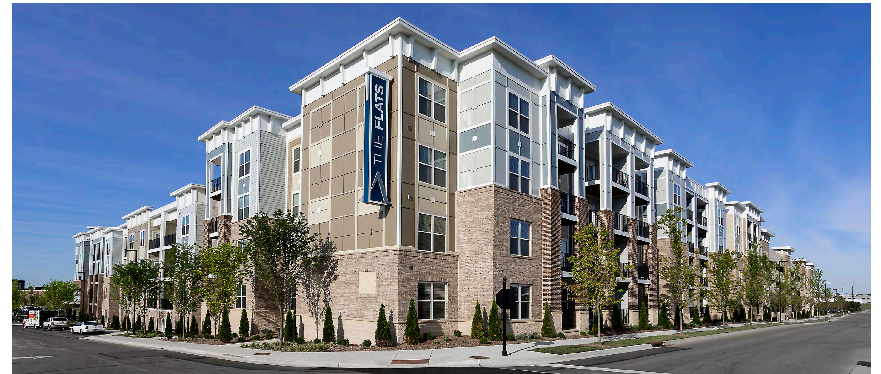
Undulating traditional architectural stacked horizontal and vertical facade elements with a rhythm of a subtle blended palette of paired masonry and cementitious panels
