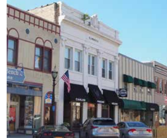
Warner Building / Built in 1909 / 83 N. Williams
