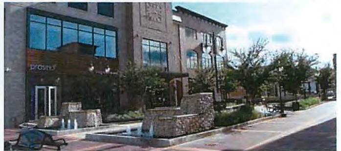
Character Image: (Top) Flex-type building; (Center-left) L-shaped building to screen loading bays; (Center-right) Stormwater detention system as an attractive and central feature of an existing business park; (Bottom) Outdoor gathering space adjacent to developments.
