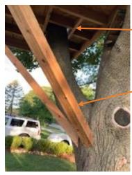
Structure solely supported by tree using 12" galvanized screw bolts through 8x8 lumber and 4x4 supports
