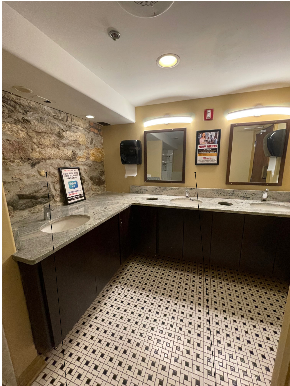
Existing stone wall, counter top, plumbing fixtures, mirrors, vanity light & vanity apron to remain
