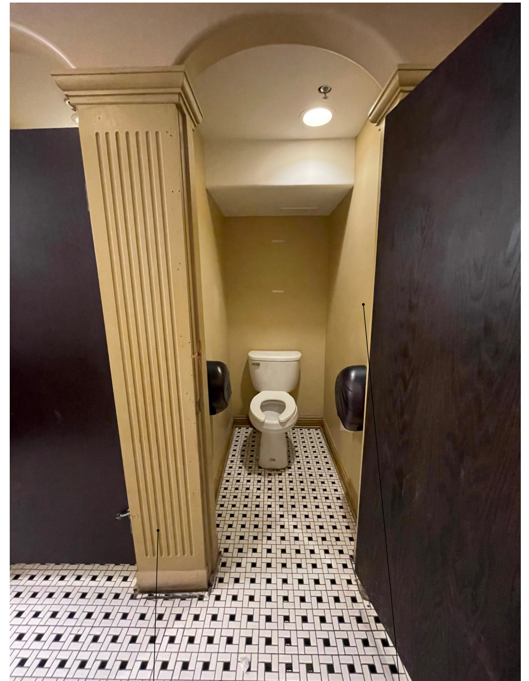
Remove toilet partition & replace w/ new stainless steel partitions
