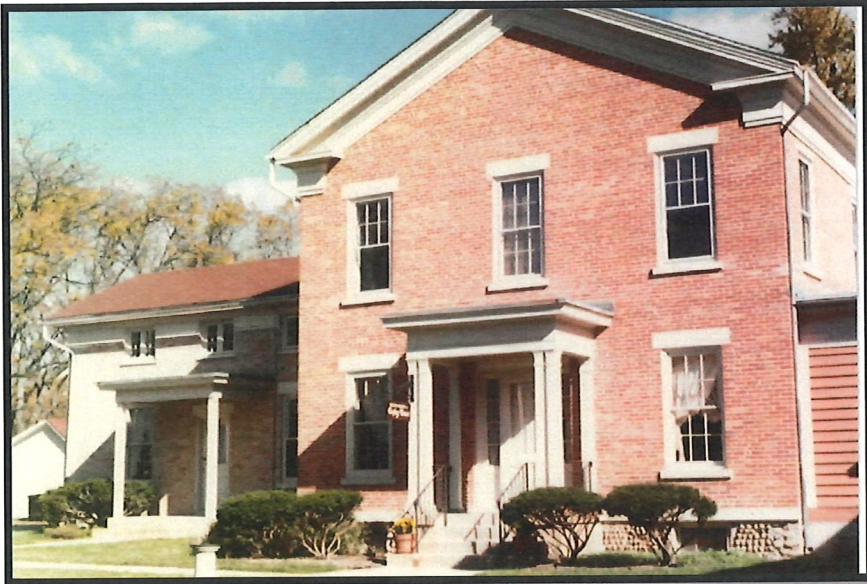
Below: Undated (circa 1980s?) photograph of Tarpley House with closeup view of cobblestone foundation.
