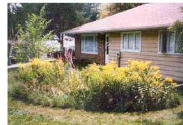
A rain garden used to mitigate residential runoff
