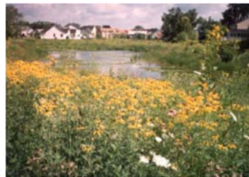
A naturalized detention basin
