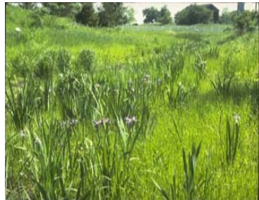
A vegetated swale
