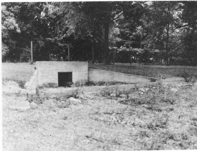
FIGURE 8 CRYSTAL LAKE DAM AND SPILLWAY
