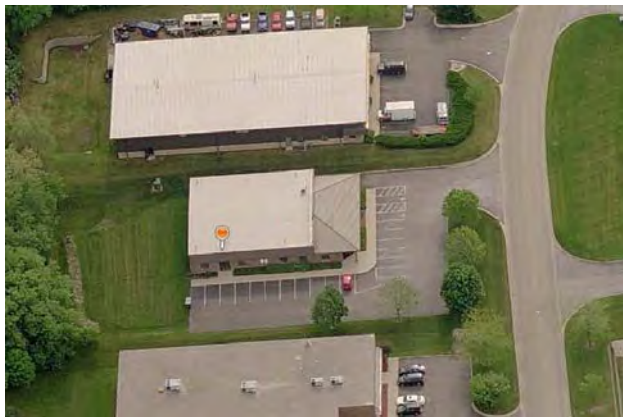
View of the surrounding area and site.
