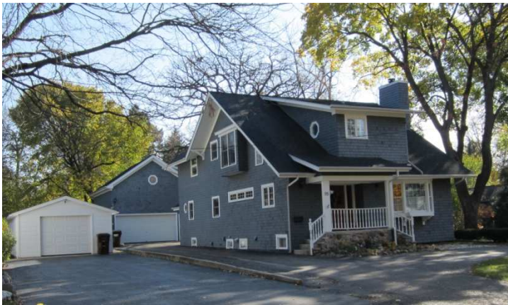
Principal and accessory structure at 95 S. Oriole St
