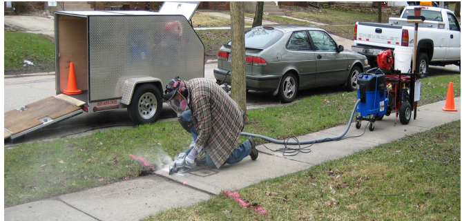
Annual sidewalk repair program
