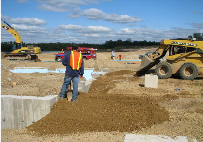
Construction of Three Oaks Recreation Area Lake building
