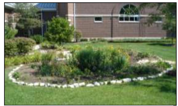
Rain garden installed to catch run-off and increase filtration at the Municipal Complex
