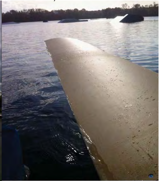
TYPICAL HDPE FLOATING DOCK / WAVEBREAK SYSTEM
