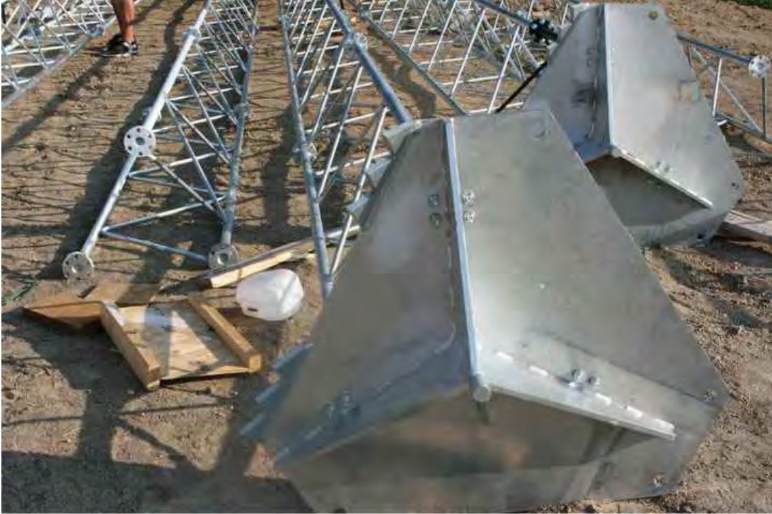
TYPICAL TOWER – BASE PLATE INSTALLED
