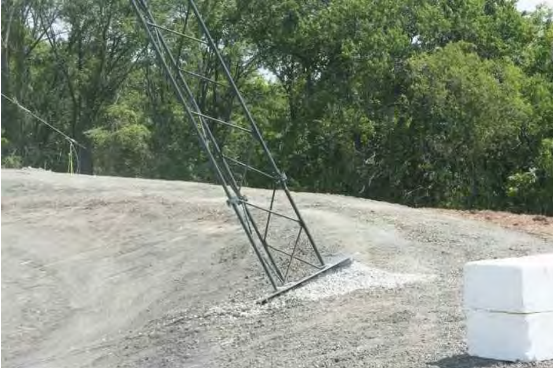
TYPICAL TOWER – BASE PLATE INSTALLED
