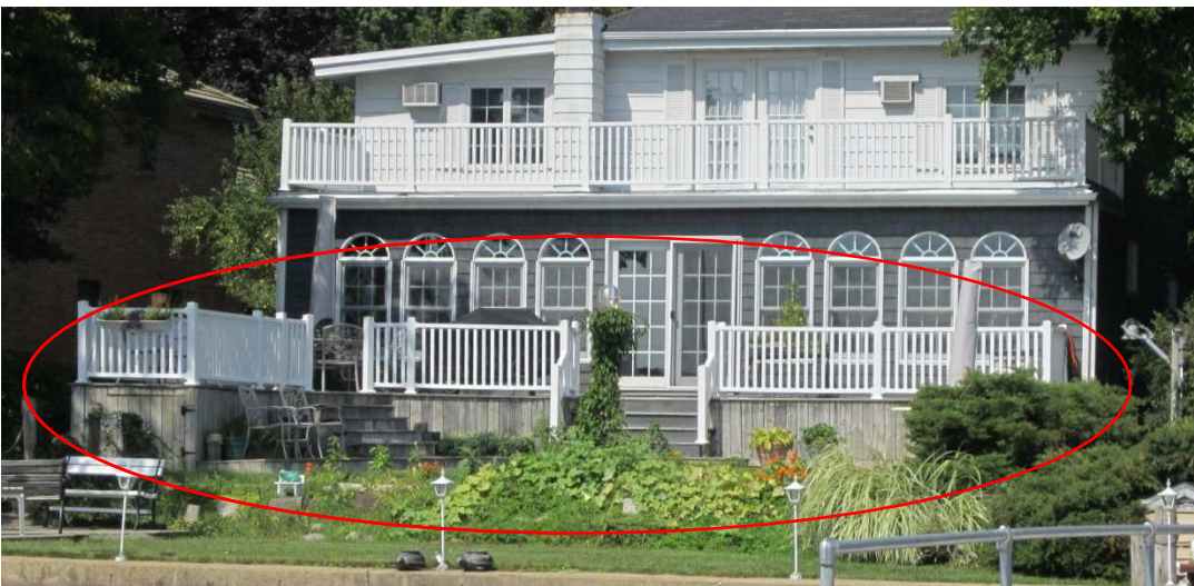
Raised deck extending from the house.
