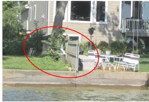
4-foot solid board-on-board fence to lake.
