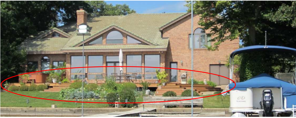
Wood deck extending out with stairs toward the water farther than permitted 4-foot encroachment.
