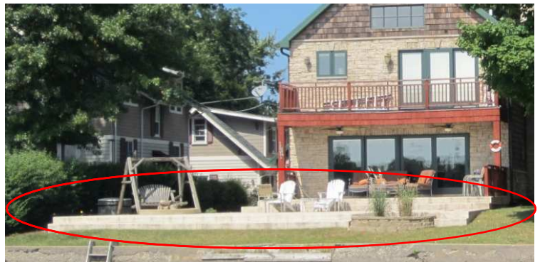
Flat concrete patio extending out near the water's edge.
