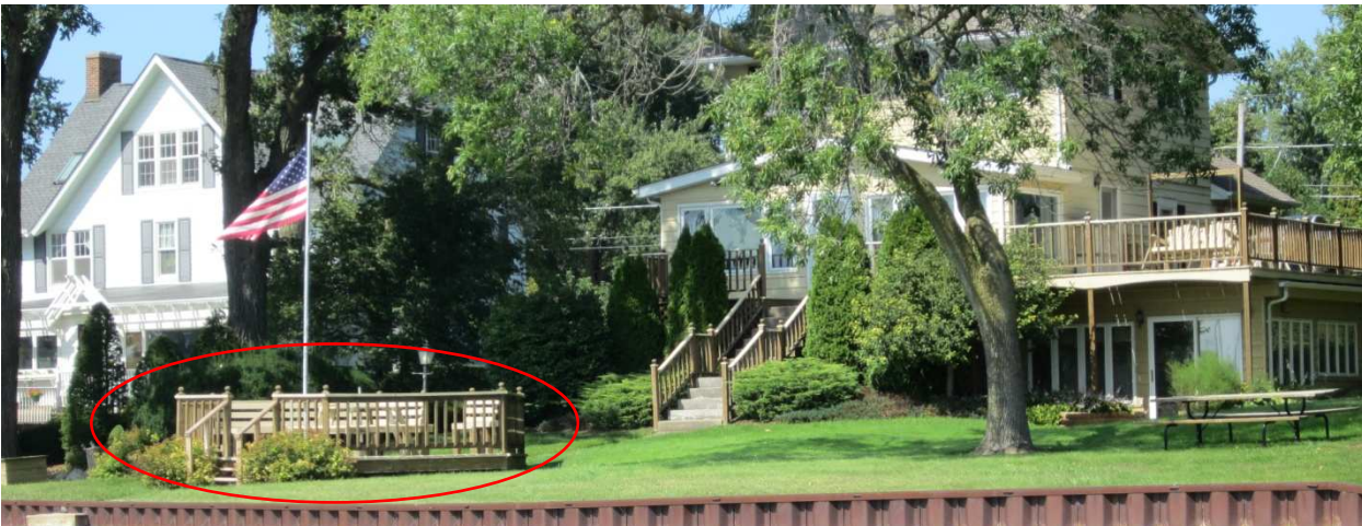
Second wood deck structure built near water's edge.
