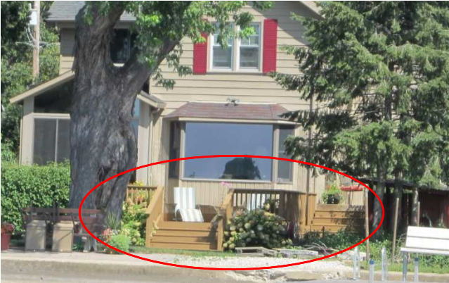
Deck extending out from the house farther than the permitted 4-foot encroachment.
