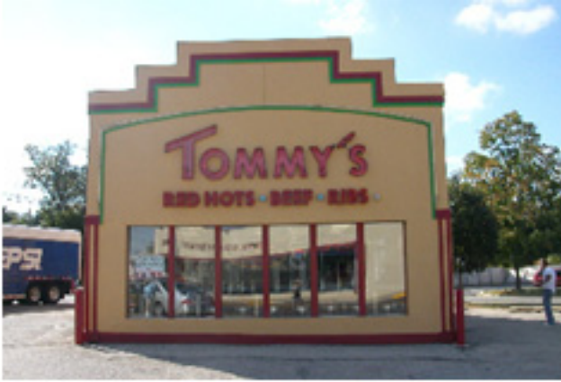
Example of building of type 2 with non-contextual elements that can be transformed.
